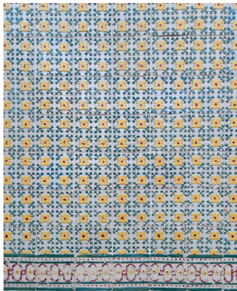
Figure 13. Azulejo on 58 Monsenhor Vieira de Castro street
